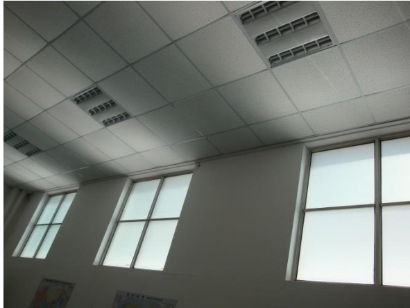
Prismatic film on the side windows
