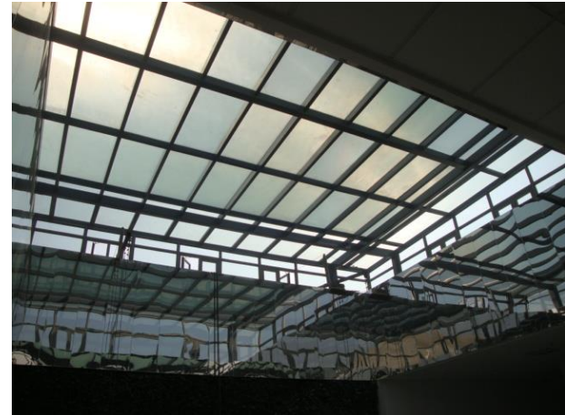
Prismatic film glazing on the atrium
