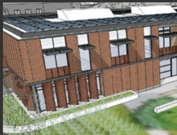
Fixed Horizontal Overhangs
