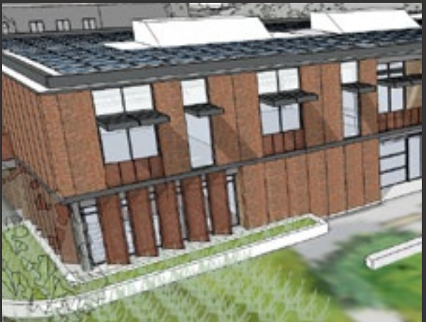
Fixed Horizontal Overhangs
